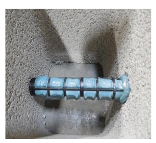
Specially sized holes in Opti-Mesh screens allow for adhesive to seep out at the appropriate location at the hollow portion of the CMU to create a better bond to the face shell.
