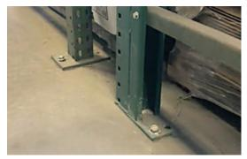
Typical low-corrosive environment — interior warehouse.
