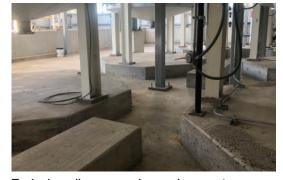
Typical medium-corrosive environment — exterior anchorage.
