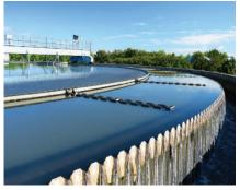
Typical severe-corrosive environment — wastewater treatment plants.
