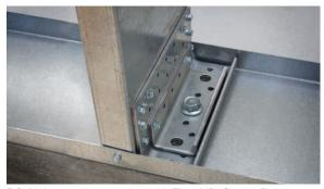
RCKW kneewall connection with Titen HD, Strong-Bolt 2 or anchoring adhesives
