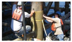
FX-70® structural piling repair and protection system
