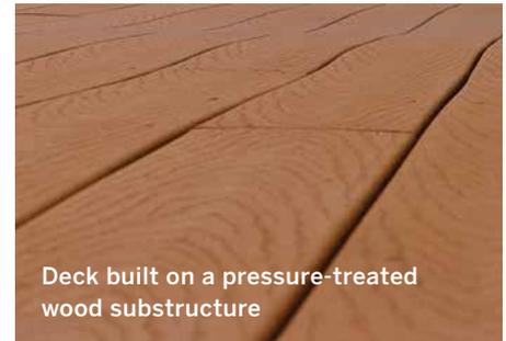
*Wood substructures split, warp and shift over time, leading to undulations in the deck boards above. The dimensionally stable steel of Trex Elevations® stays in place, creating consistently flat decking. To watch a video demonstration, visit [trex.com](https://www.trex.com)*
